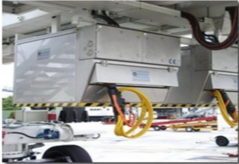
Bridge Mounted Cable Coiler
