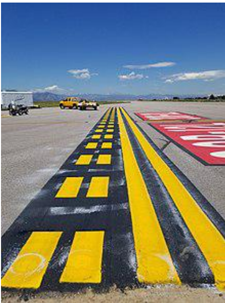
A newly painted Runway Holding Position Marking at Rocky Mountain Metropolitan Airport (KBJC)
