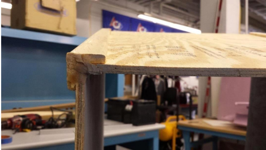
Wooden corner guard connecting plywood sides of diverging section
